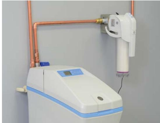
Whole home filtration connects to your home's main water line to reduce sediment, scale, dirt and rust.
